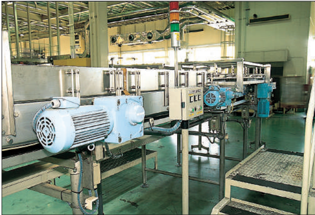
Conveyor lines in breweries
